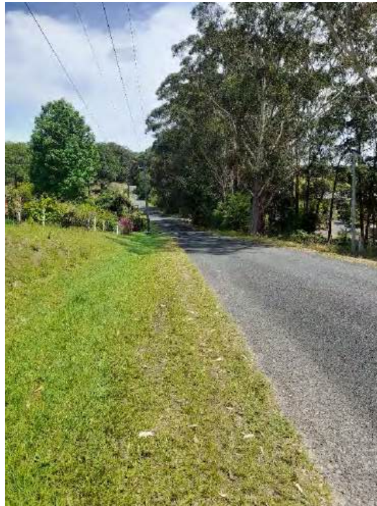
Proposed access at 89 Sugarmill Road looking west. Proposed Lot 170 (Sight distance >90m)
