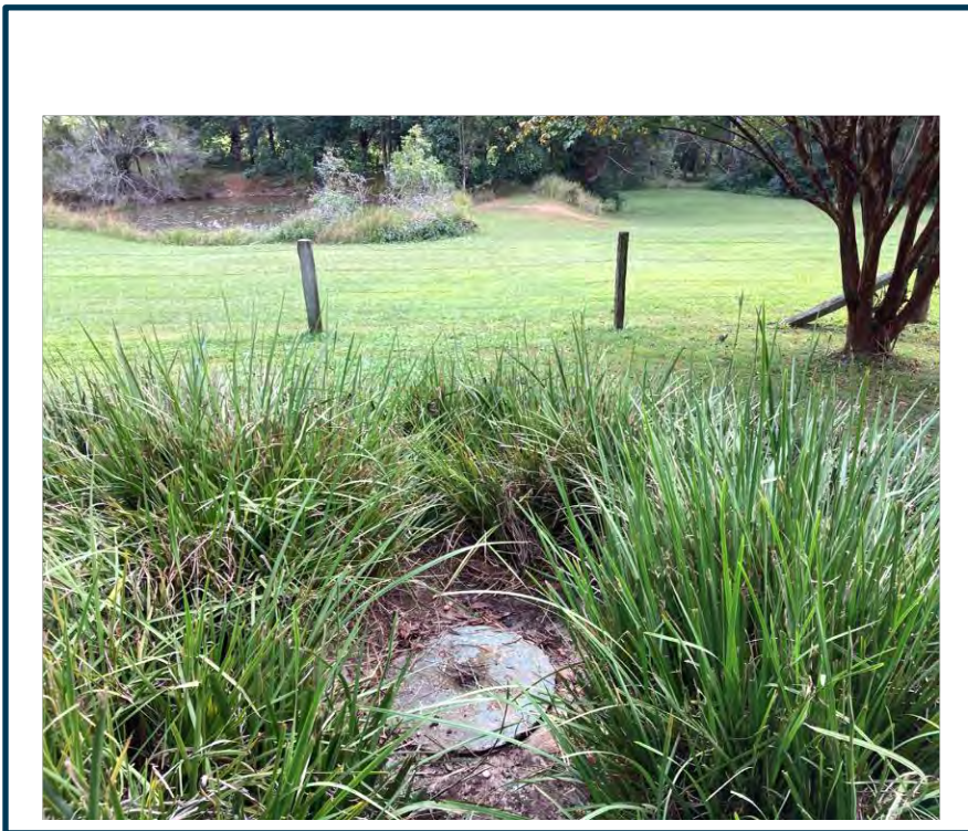
Photograph 3 – The existing Septic tank on Lot 120.
