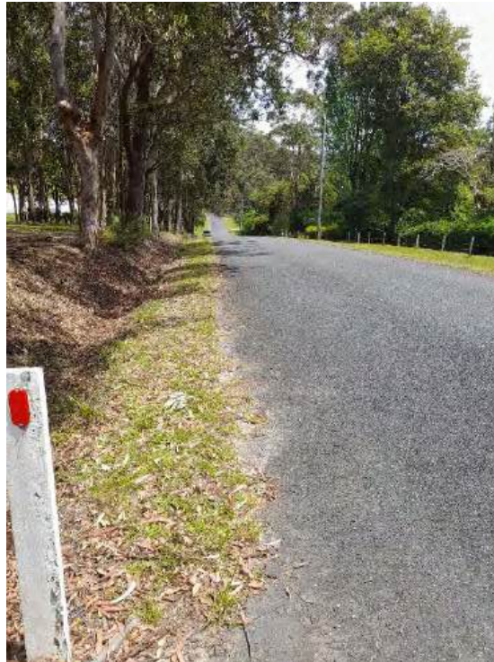
Existing access at 35 Sugarmill Road looking west. Proposed Lot 910 and 911 (Sight distance >90m)
