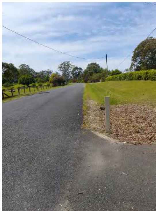
Existing access at 35 Sugarmill Road looking east. Proposed Lot 910 and 911 (Sight distance >90m)
